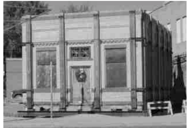
The old Vananda Bank building sitting on its new foundation will become the " Palomino Mercantile "
